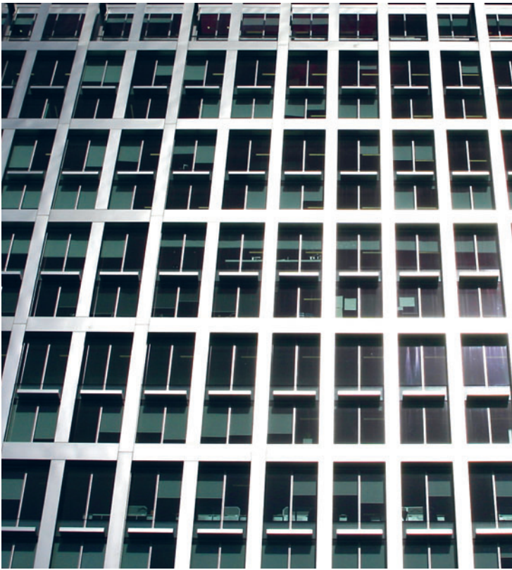
5 Aldermanbury Square, London, 2005 Arquitecto Eric Parry Architects; Fachada Lindner-Schmidlin UK
