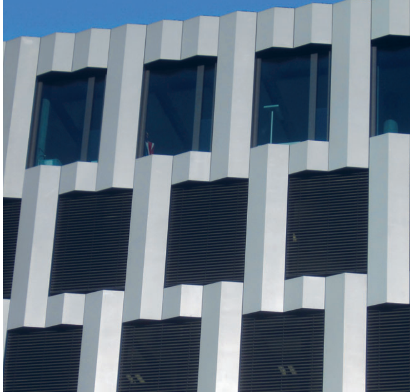
Office Building Zurich West, Zurich, 2013 Fachada Yuanda Europe
