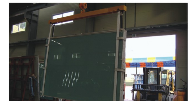
One crate lifting work with crane system
