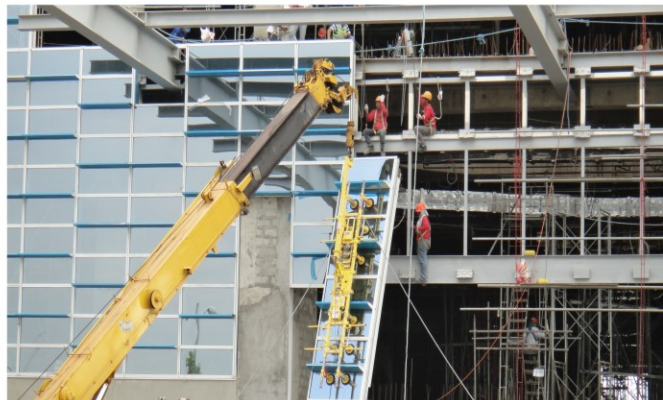
Crane with lifter
