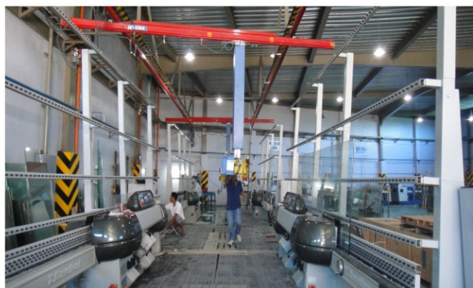
Vertical grinding machine with lifter
