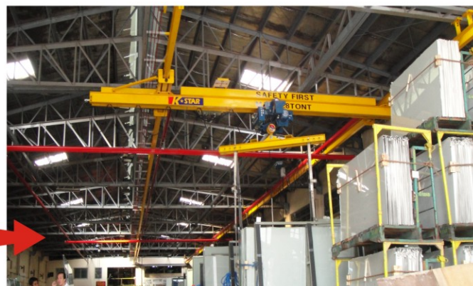
Suspension Crane (After)
