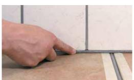
Backfilling the joint with OTTO PE-B2
