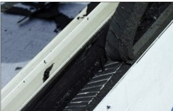
Figure 31: Example with black SG joint - Good adhesion.
