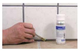
Possibly prime the adhesive flanks with the appropriate OTTO Primer or Cleanprimer with a soft paintbrush on absorbent substrates or with a soft cloth on non-absorbent substrates.
