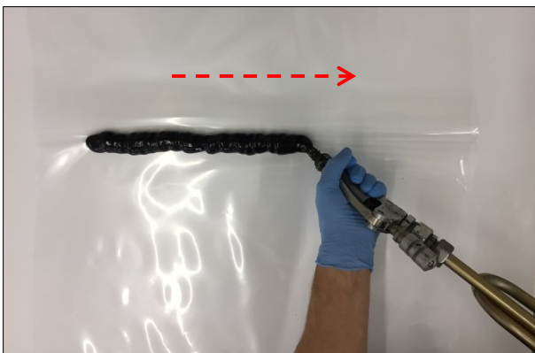
Figure 6: Apply the bead in the fold direction
