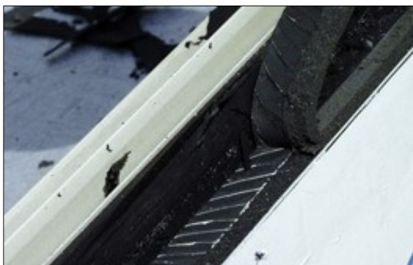
Figure 31: Example with black SG joint - Good adhesion.
