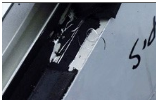
Figure 32: Example with black SG joint - Adhesion failure.
