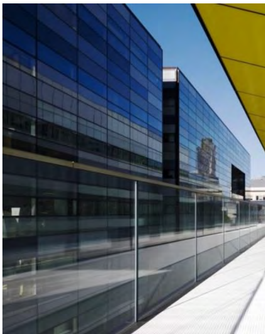
Picture 1: Glass embedding in postless guard rail
